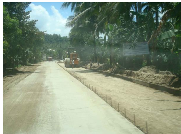
b. Compaction of sub-base layer
