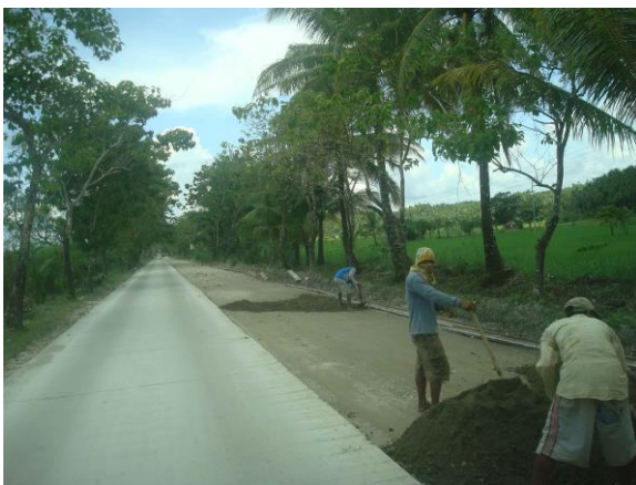
a. Manual laying out of sub-base material
