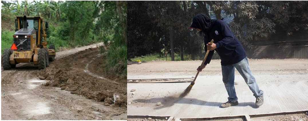
a. Rehabilitation along local road Source: cotabatoprov.gov.ph
