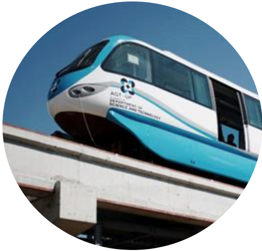
Automated Guideway Transit (AGT)
