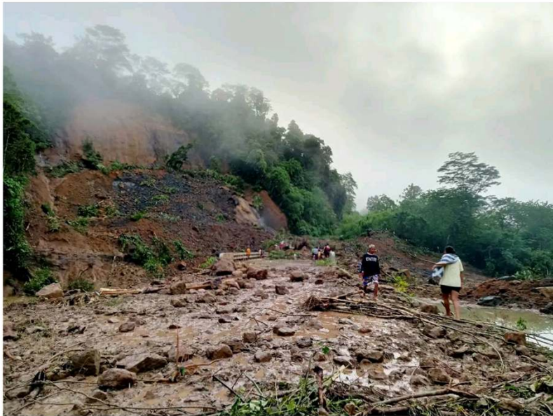
A bridge in the remote Mahayahay village in San Luis, Agusan del Sur is nearly covered by debris in this photo from a netizen's Facebook post.
